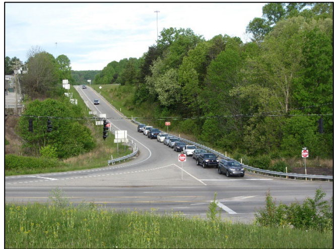
Traffic Queueing on the I-64 EB Off Ramp
